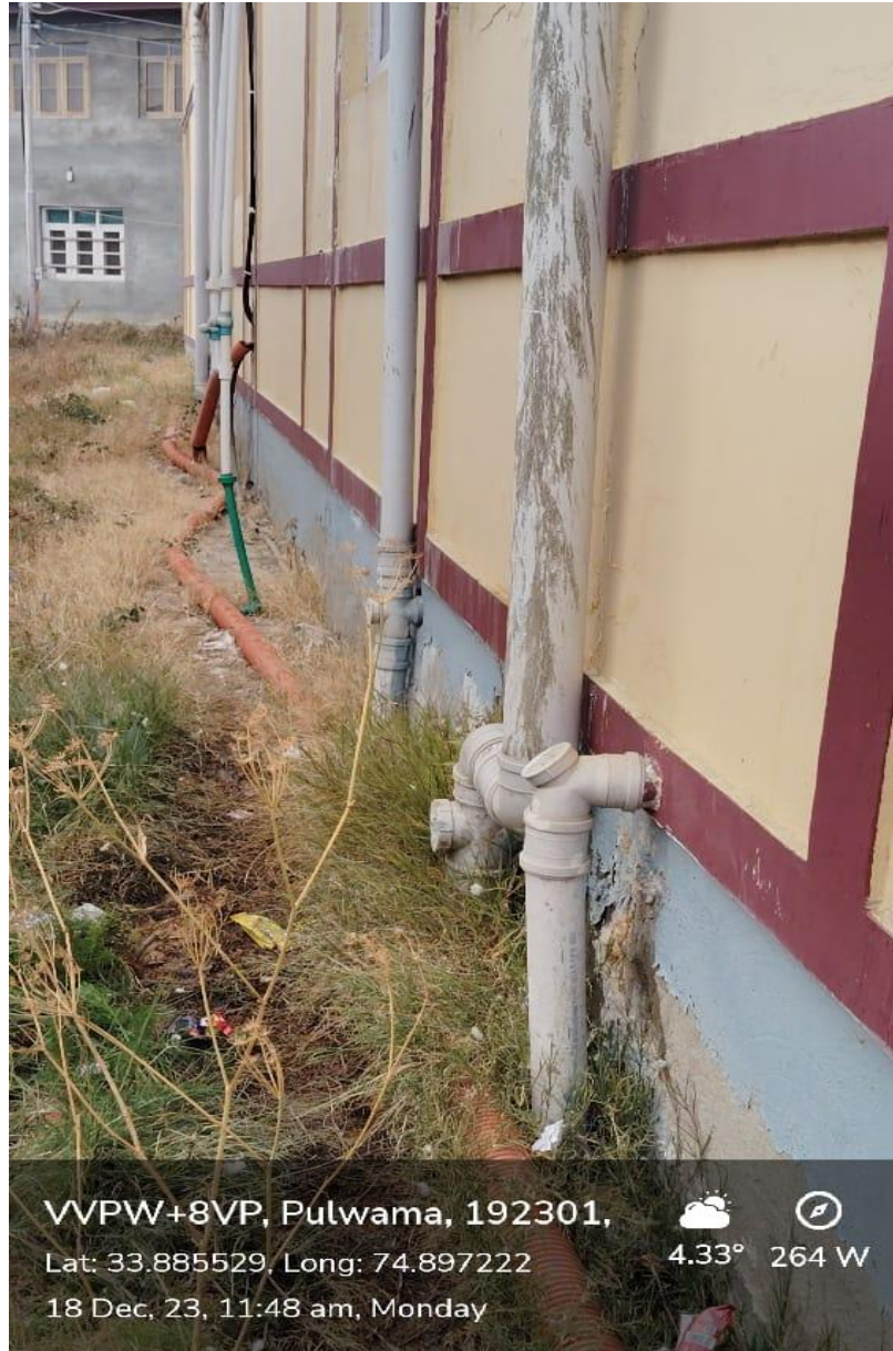
Sewage outlets towards underground
